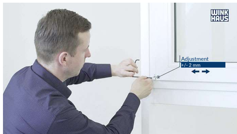
Horizontal adjustment of the frame-side hinge
