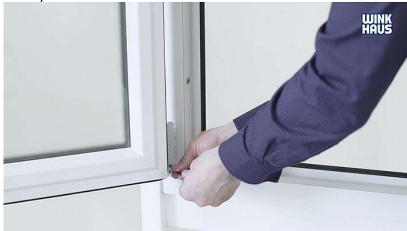
Adjustment of the holding force on the left-hand casement
