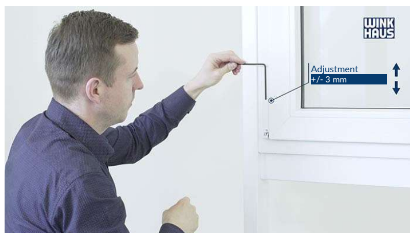
Height adjustment on the casement hinge
